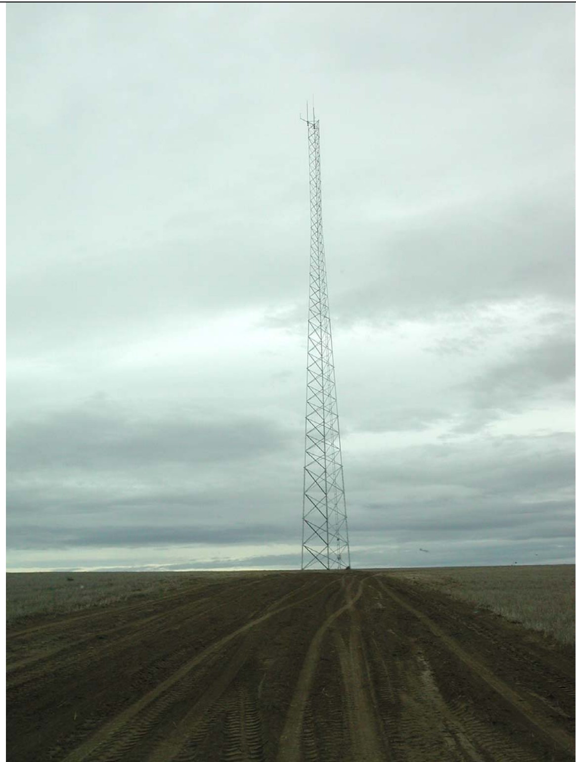
Figure 4. Lattice unguyed meteorological tower at the Nine Canyon Wind Project.
